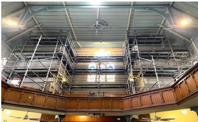
Scaffolding – Leigh Memorial northern end.
