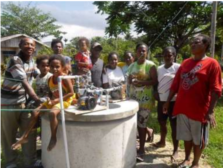
Construction of well completed – and a happy community
