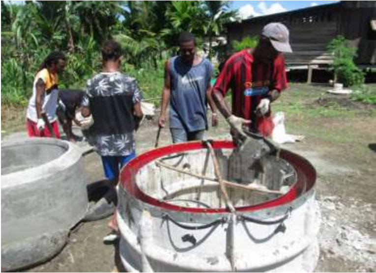
Well under construction in West Papua
